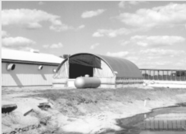
◆ Hislop Farms constructed a hoop house for composting mortalities.
