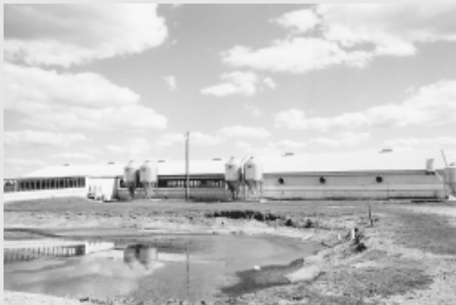
◆ Hislop Farms has a 500,000 gallon clay-lined earthen basin for manure.
