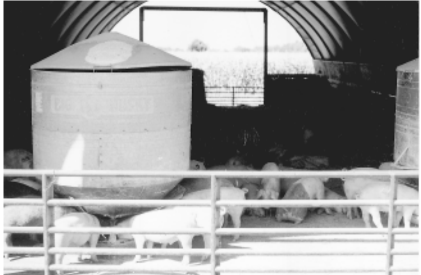
◆ A 30' x 72' hoop structure can accommodate more than 180 hogs.
