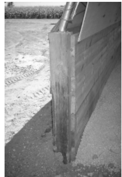
◆ Hoops are built on a lime or gravel base and sloped away from the feeding area.
